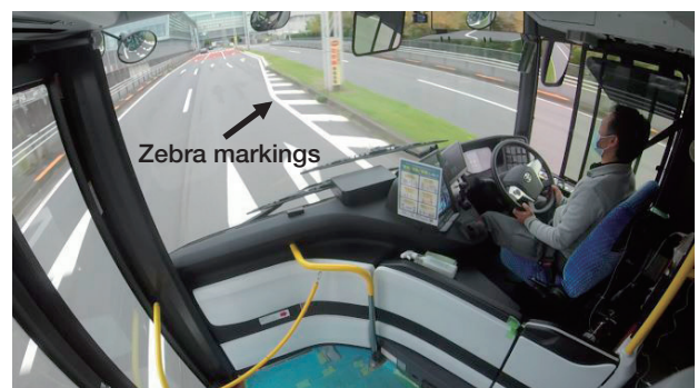
Photo 1 Zebra Markings before Right-Turn Lane
