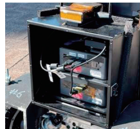
Fig. 5 Main ECU (Inside ECU Box)
