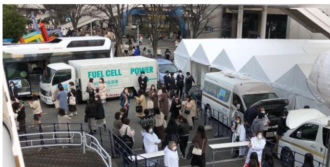
Fig. 48 Example of Electricity Supply at Concert Venue
