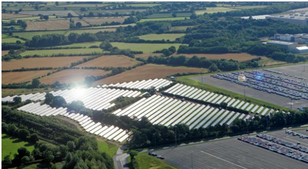
Solar Panels in TMUK
