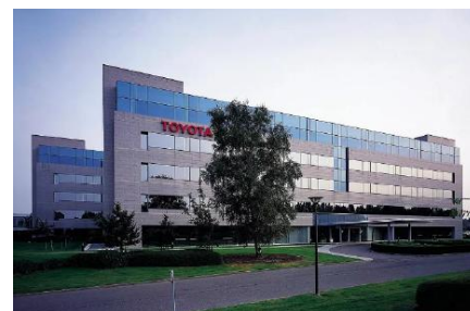
TME Headquarter Building
