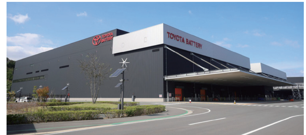
The Arai Plant (operational in 2024) where the ceremony was held
