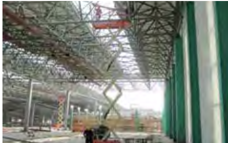
China: Check on construction sites
