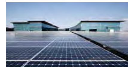
TMNA's new North American Headquarters Campus (solar panels installed on the building)
