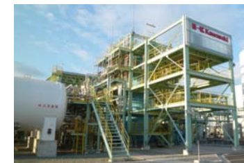
Hydrogen liquefied from gas at -253°C (1/800 volume)
